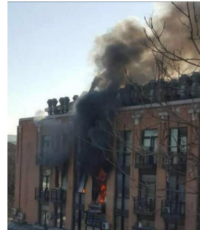
Explosion occurred in Tsinghua University when doing testing using hydrogen in 2015
