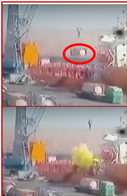
Figure 1. Cable fails while lifting a Chlorine isotainer
